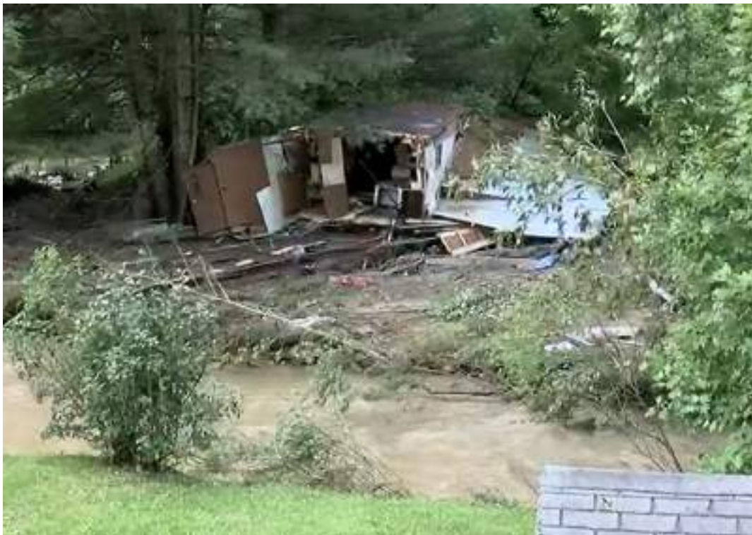
Figure 644: Mobile Home that was Destroyed during the July 2022 Flood Event in Bandy, VA 51
