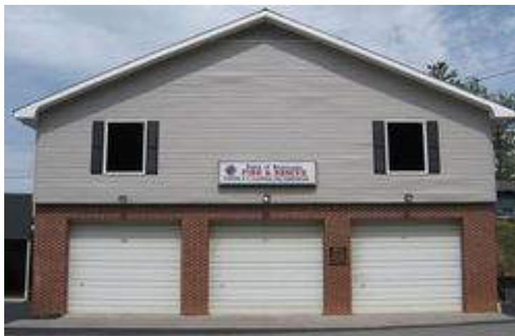
Figure 75: Richlands Fire-Rescue Station 3
